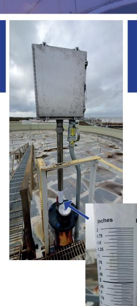
MTG "Multi-function Tank Gauge" measures both the fumes and the product in addition to reference point movement.
